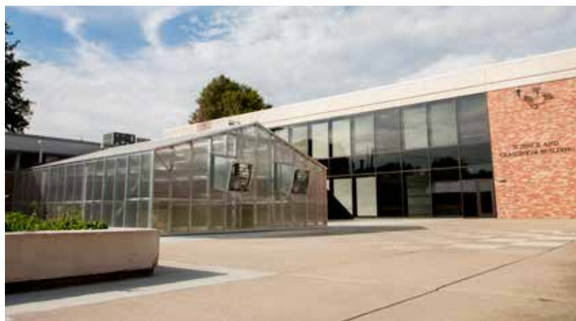
The Elings Science and Classroom Building received some summer updates. The old greenhouse, previously on the east side of the building, was demolished and a new greenhouse, approximately 720 square feet, was constructed in the Elings courtyard. Other renovations included complete remodels of two classrooms, updates to two other classrooms, and new ceiling tiles and LED lighting throughout several areas of the south wing of the building. PHOTO: LACIE SIBLEY '07
